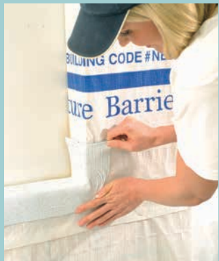
Begin by installing the sill – our self-adhering membranes protect the sill from moisture damage. All caulking must be fully cured before installation.
