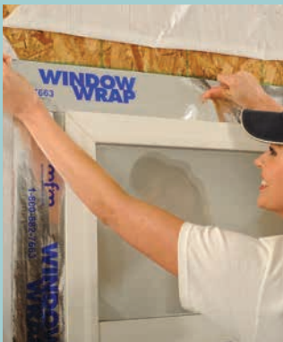
Adhere WindowWrap® to the header flange and directly to the house sheathing. Head section must extend beyond the jamb sections for proper waterproofing.
