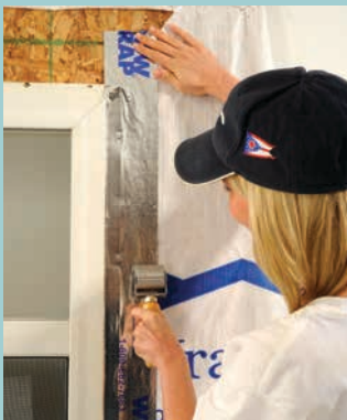
After setting window, adhere vertical sections over the side flanges and to the shear wall or house wrap. Firmly roll with a hand roller to ensure good adhesion.
